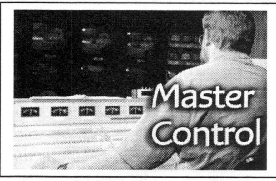
The Master Control Switcher (the board with all of the buttons) is the piece of equipment that determines what goes to air. Through most of the day programs and commercials are fed to us from CTV in Toronto via a fiber optic line, through this switcher, and out to transmitters.
